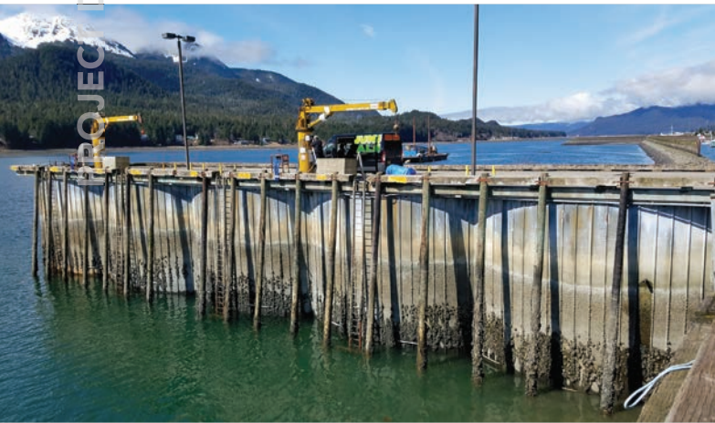
Figure 5 – (above) Fender pile and bull rail construction on south side of existing crane dock; (right) Existing Crane; (below) North side of the rubble mound breakwater where the new dock face will be constructed.
