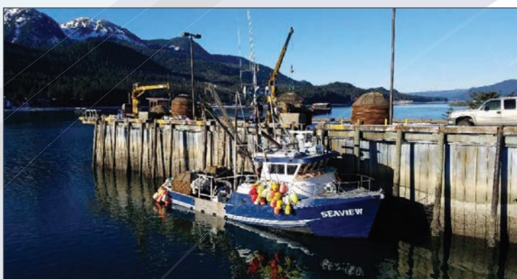
Figure 12 – Vessel Offloading Goods at Existing Crane Dock
