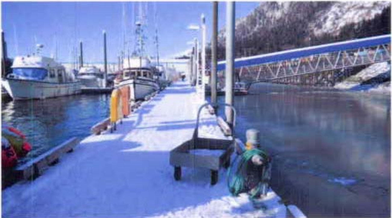
Harris Harbor loading zone & sales area.
