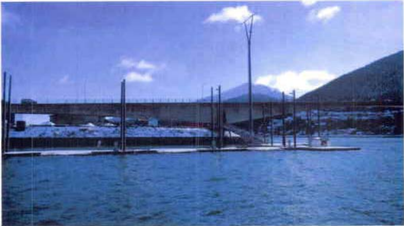
View of existing float at Bridge.
