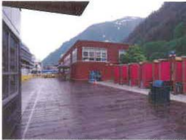
Dock under rear of Tram building.
