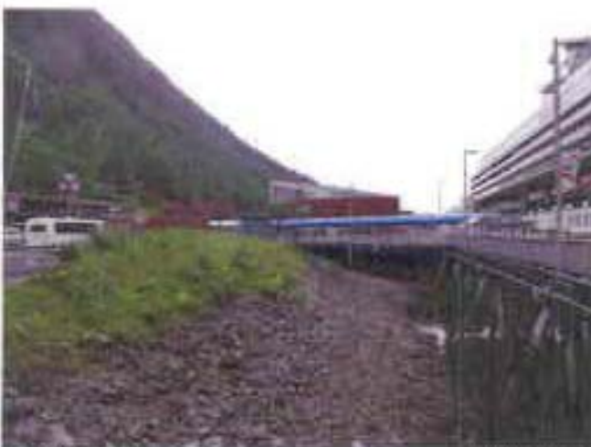
Typical shoreline nearby
