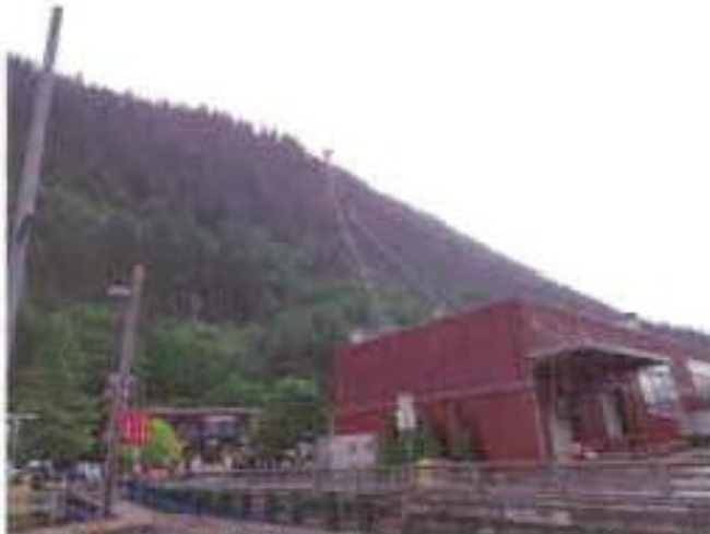
Rear of building facing the channel.
