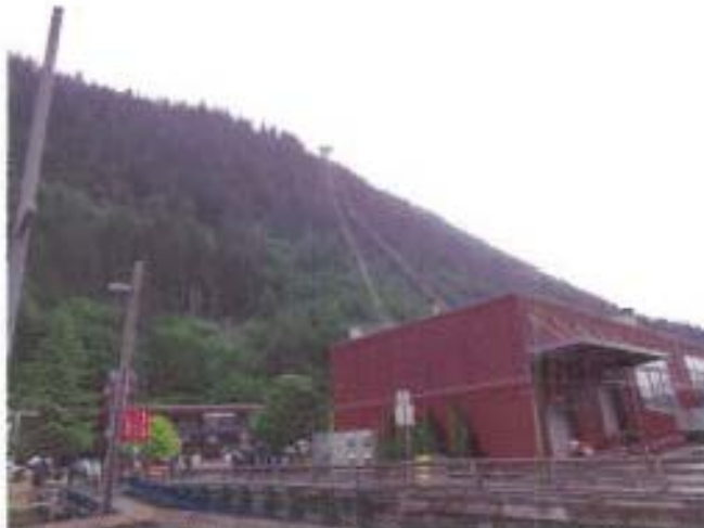
Rear of building facing the channel.
