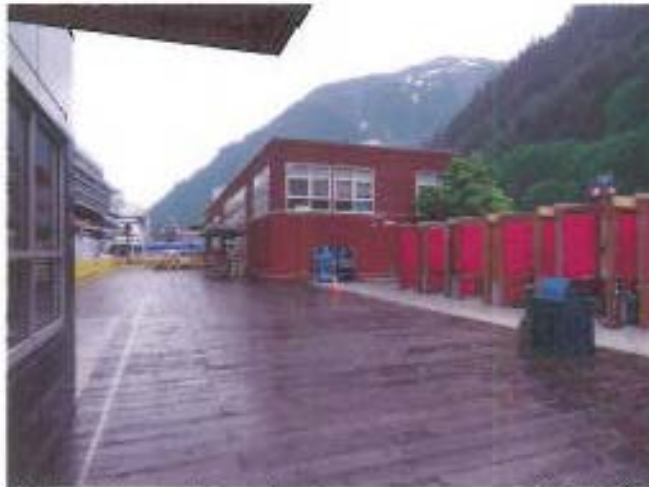
Dock under rear of Tram building.
