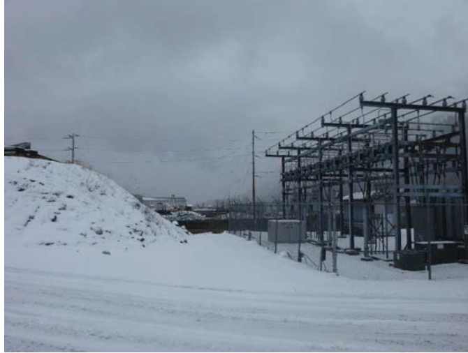
Access to subject site from State ROW.
