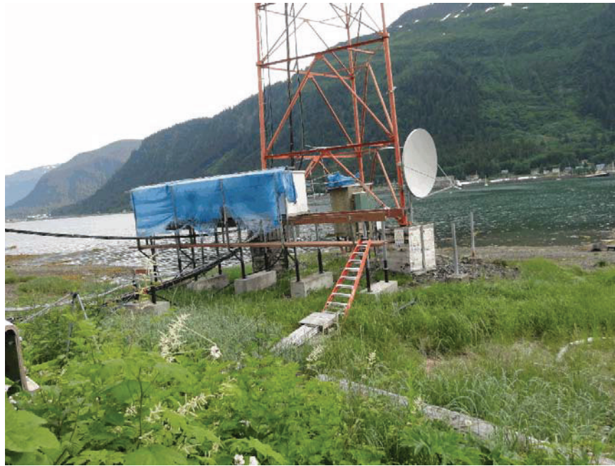
Tower on subject land.
