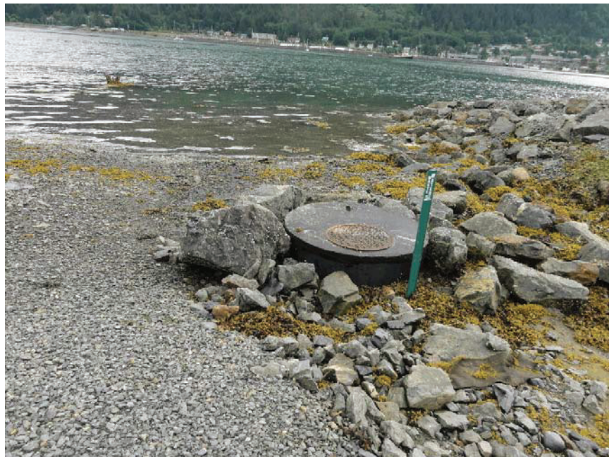
Sewer noted at meander line.
