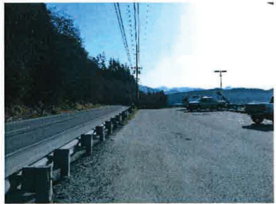
ENCROACHING PARKING AND GLACIER HIGHWAY FRONTAGE 040612_0891
