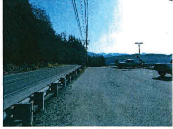
ENCROACHING PARKING AND GLACIER HIGHWAY FRONTAGE 040612_0891
