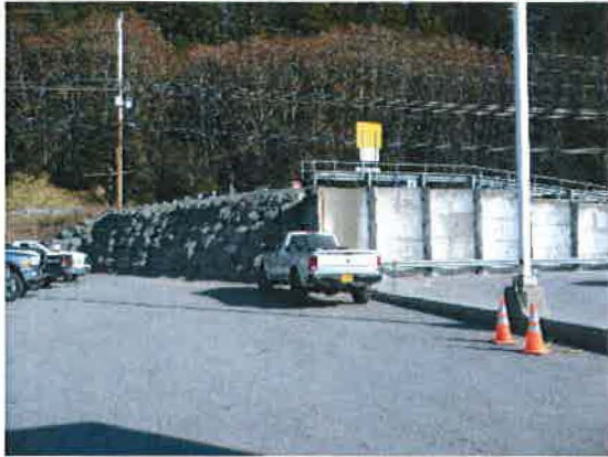
NOTE ATS 1170 BULWARK DEVELOPMENT 040612_0916
