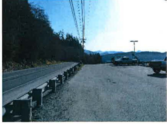
ENCROACHING PARKING AND GLACIER HIGHWAY FRONTAGE 040612_0891
