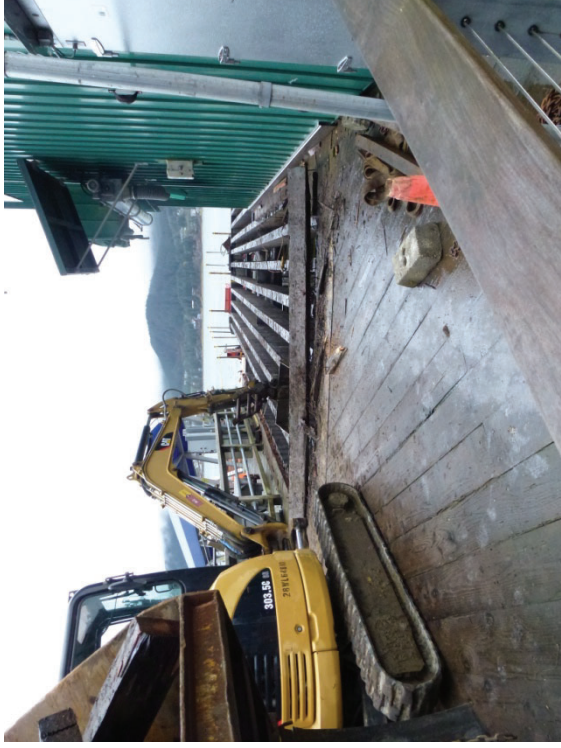
Demolition of decking
