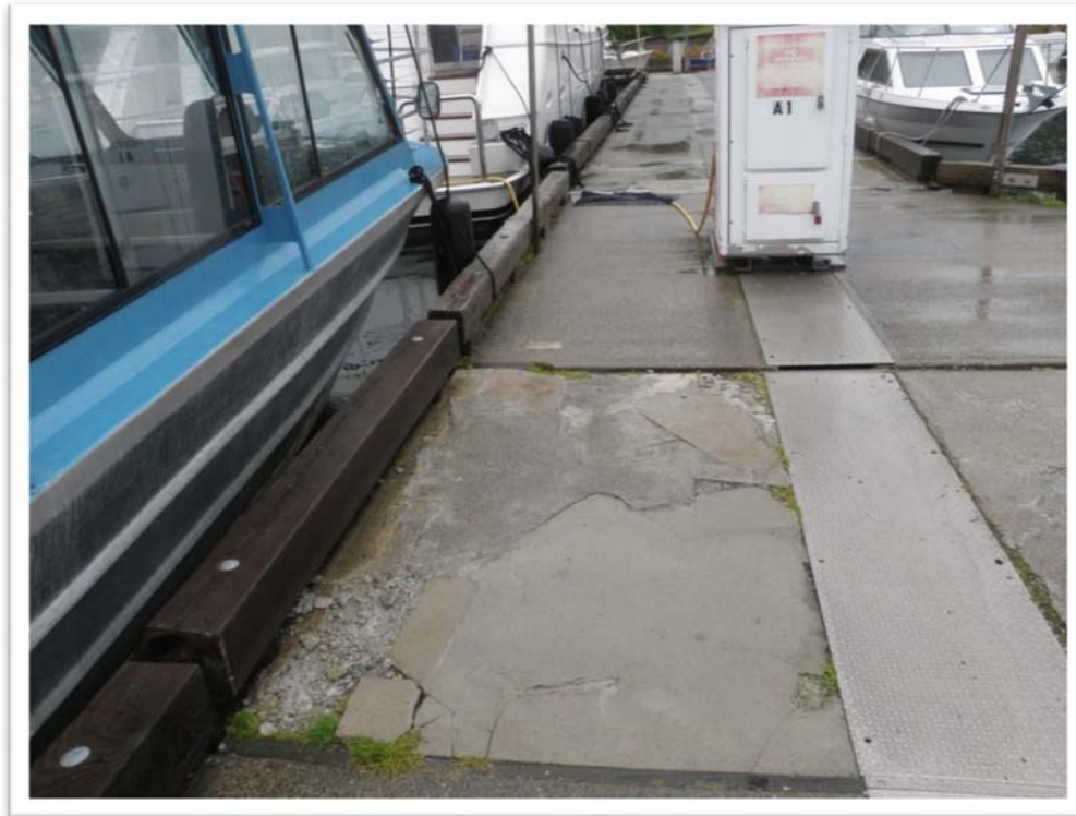
Figure 3: Previous Damage to Float Deck Prior to Failure (Photo taken in 2011)
