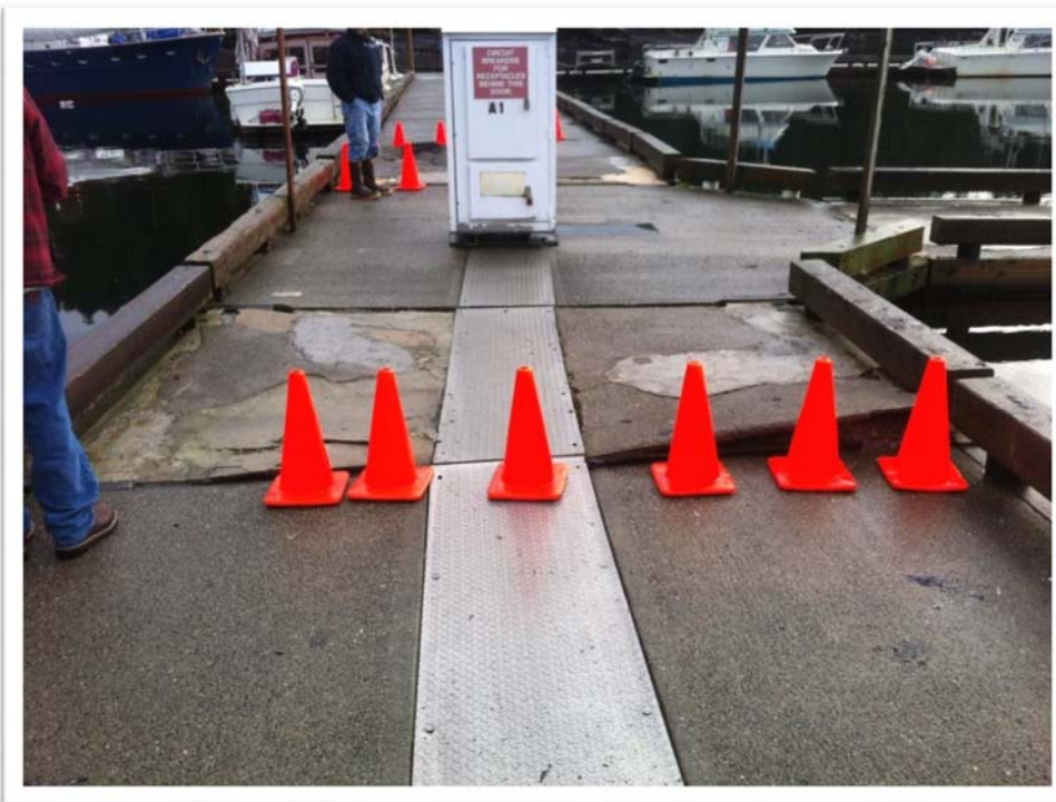
Figure 2: Crushed Float Module #2
