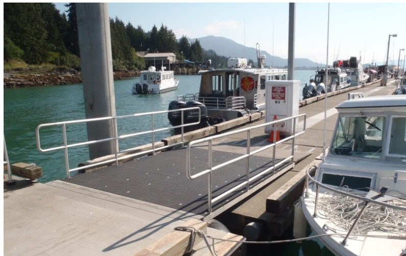
FIGURE 2 TRANSITION RAMP - 2 TO EXISTING CONCRETE DOCK
