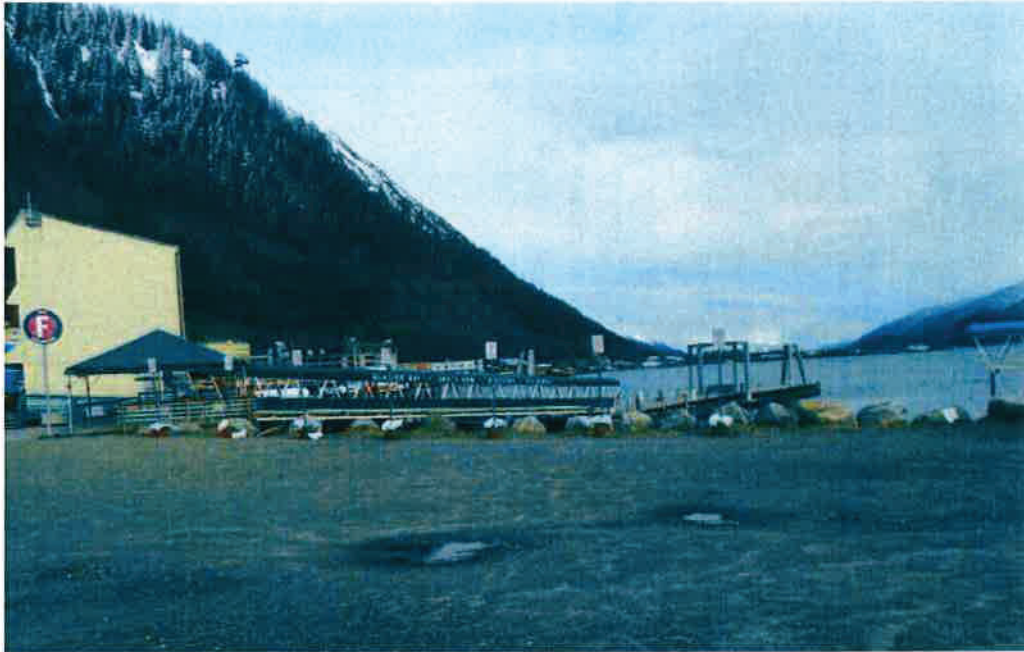
PHOTO 1 - FILLED PARCEL A & B LOOKING EAST
