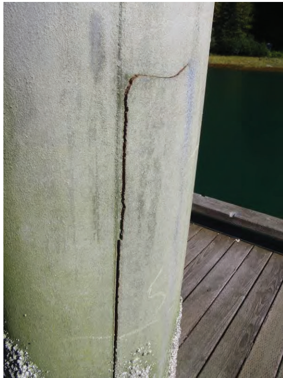
Split pile M6 on main float.
