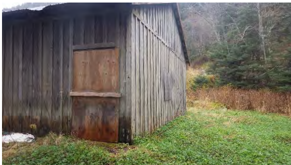
South end from west
