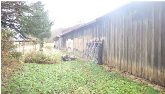
West wall from south end
