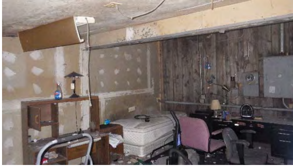
East side mechanical room with living quarters
