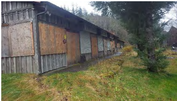
West wall from the north end
