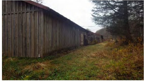
East side from south
