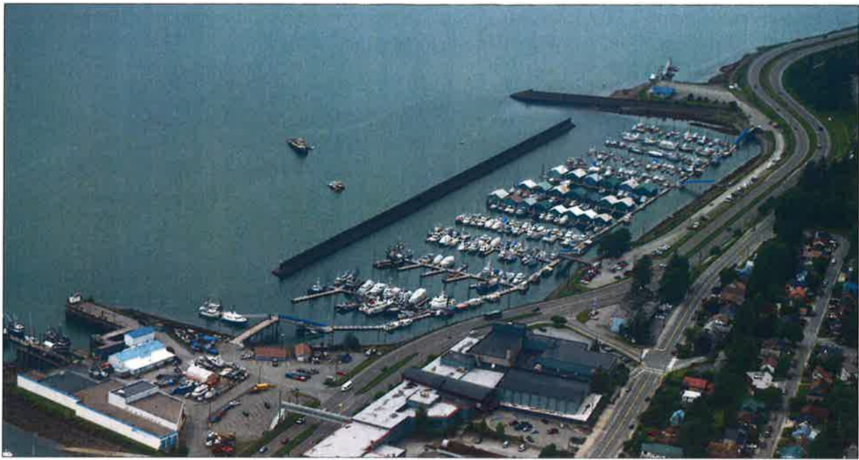
Figure 6. Aerial view of Aurora Harbor, Juneau (USACE 2017).
