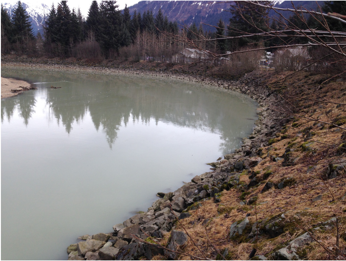
Figure 3: Existing riprap near Postal Way
