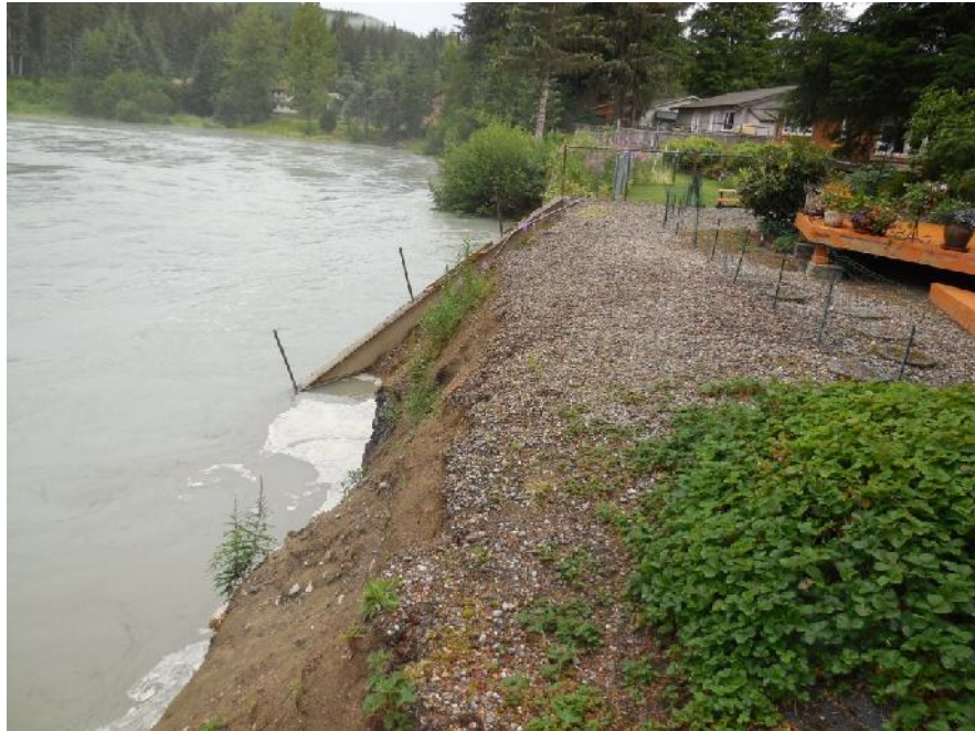
Staton residence riverbank looking upriver 2016
