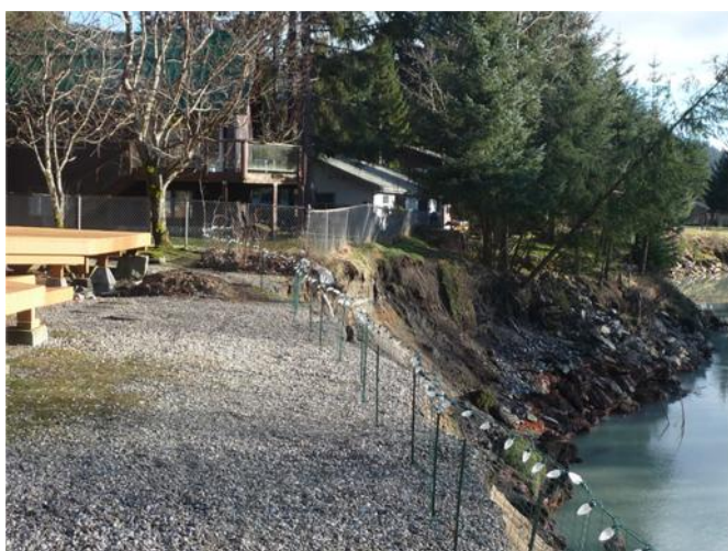
Property line looking southeast
