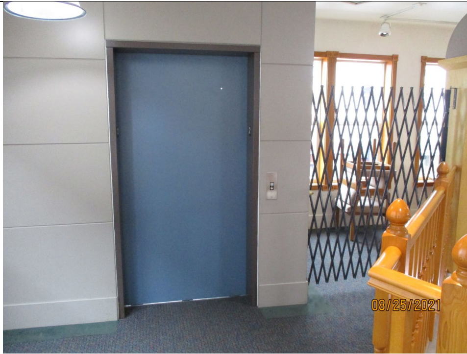
Elevator on 2 nd floor
