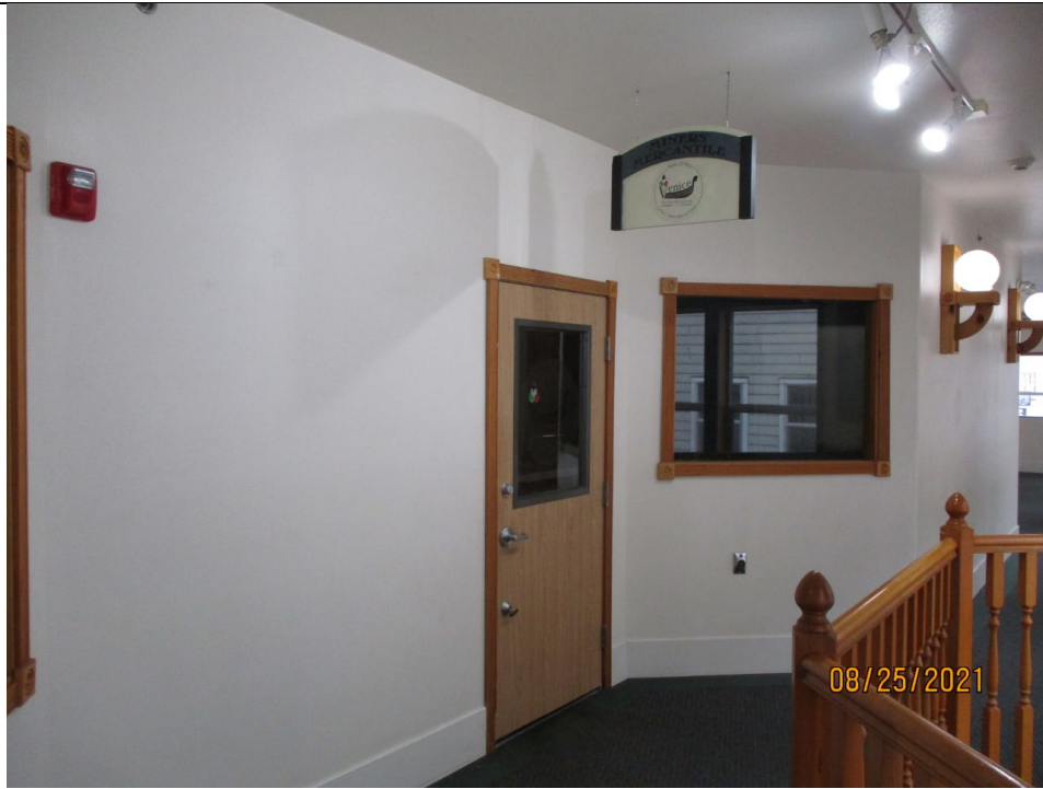
Office space on 2 nd story
