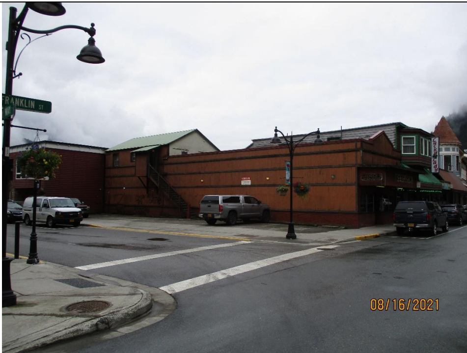
From adjacent corner
