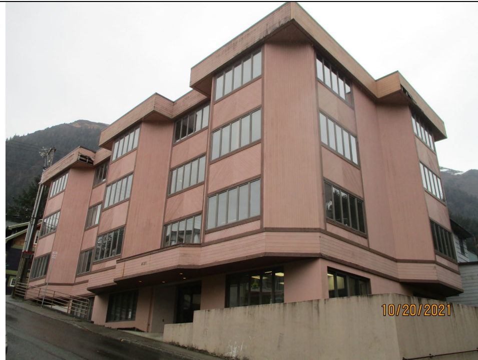
Front right from N Franklin St
