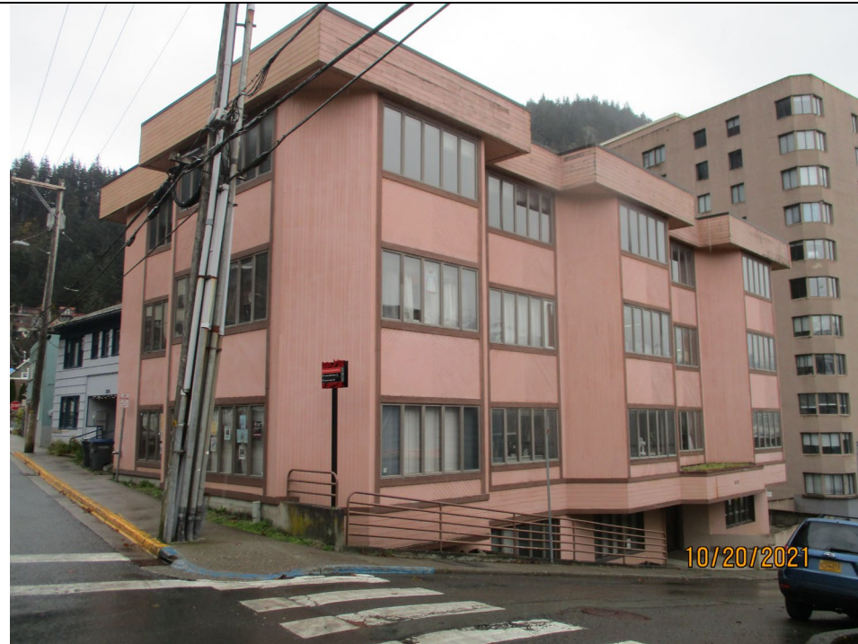
Front left from corner of N Franklin St & Fifth St
