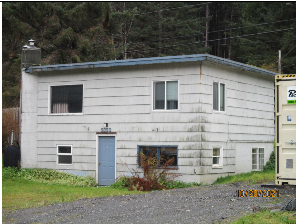
Back looking toward highway
