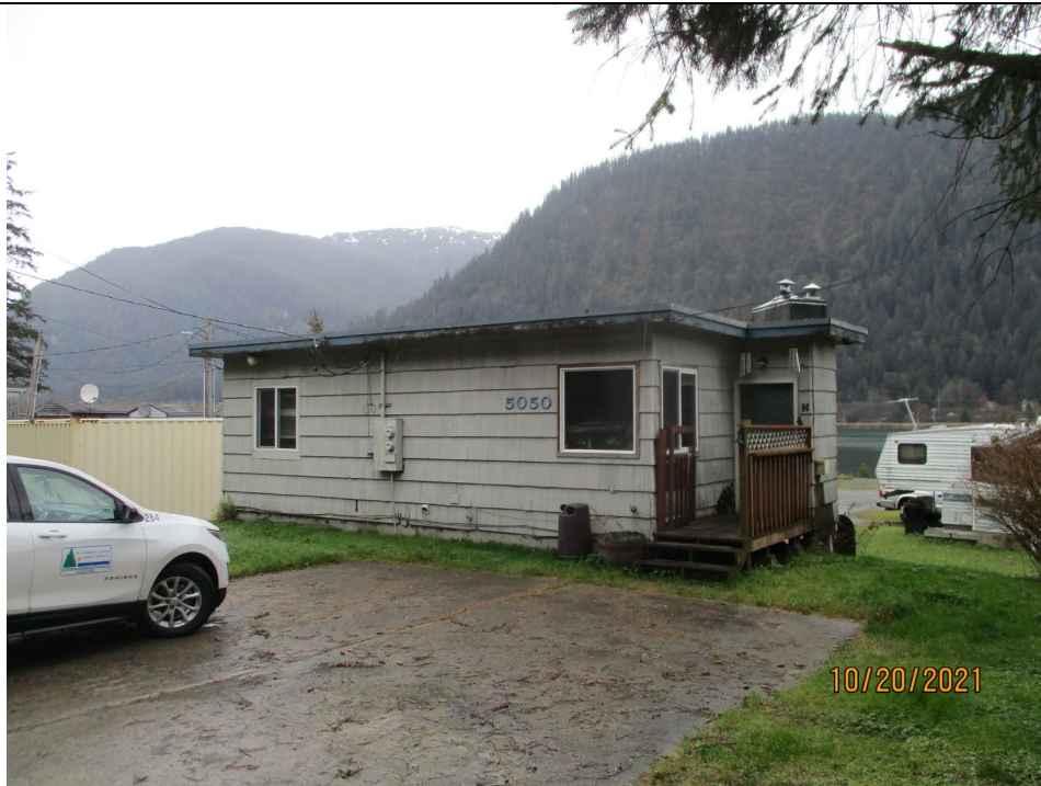
Front right from highway
