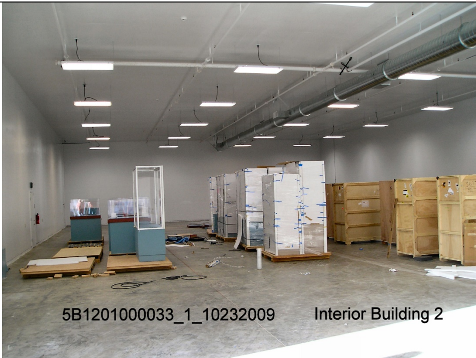
Building 2 – 2009 Interior photo
