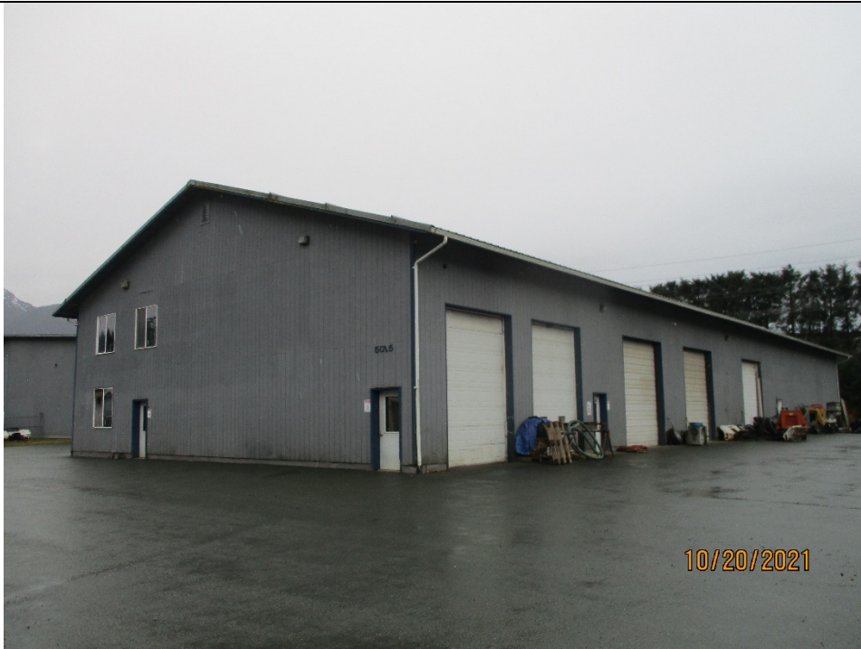
Building 2 – Front right, mezzanine office
