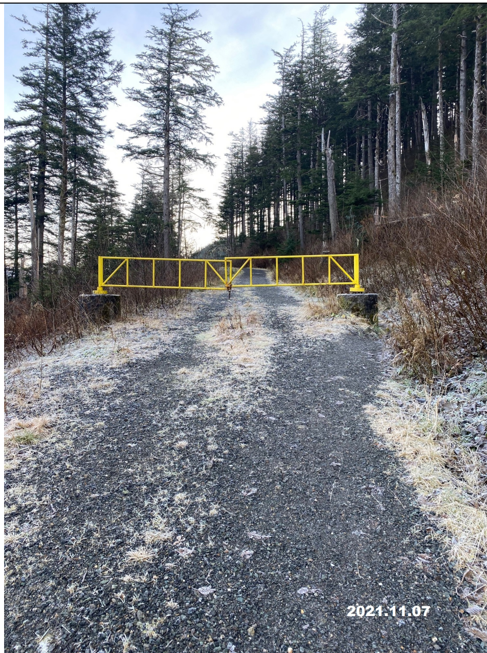
Gate at Access Road from John Street
