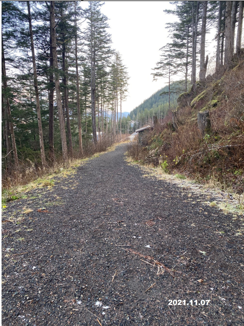
Access Road through CBJ Parcel
