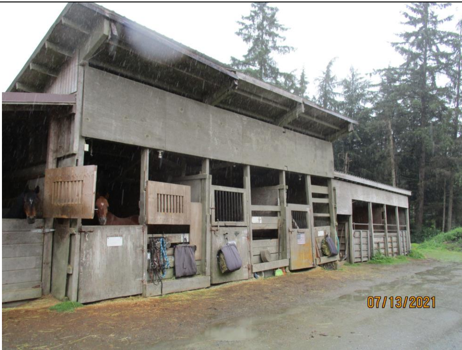
Misc storage building/ horse stalls
