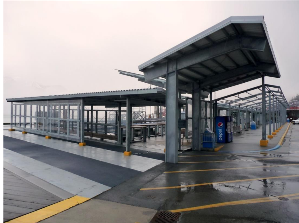
Bus passenger waiting area
