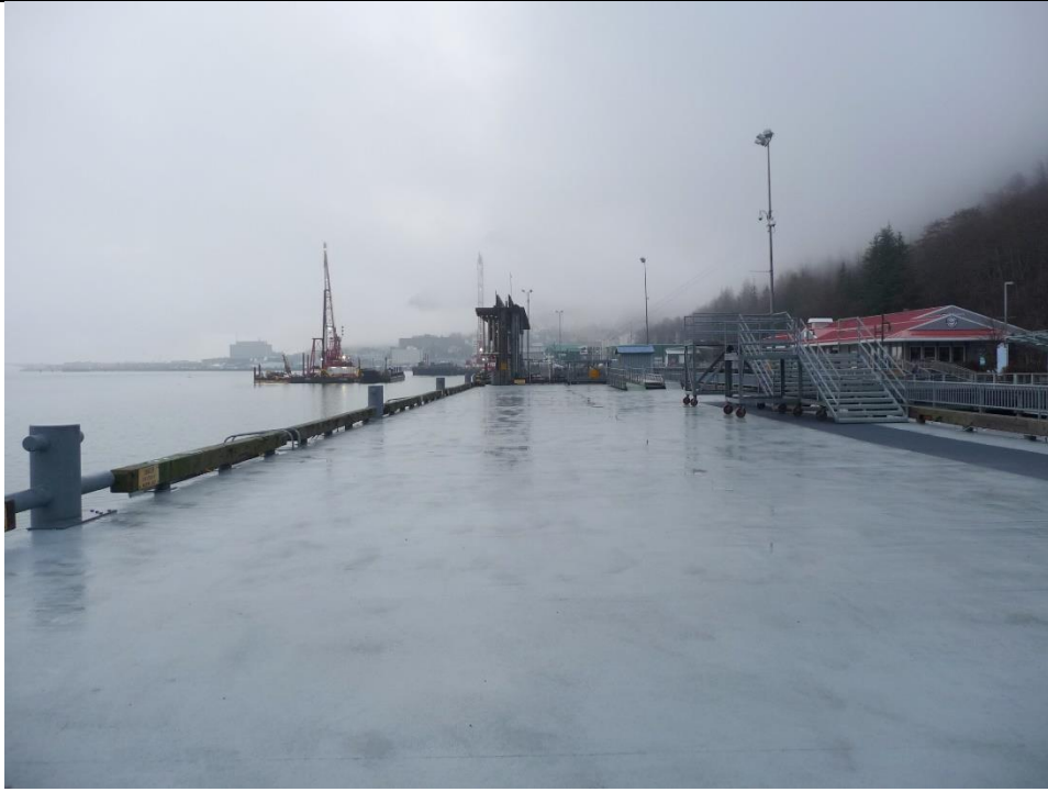
Dock structure – Looking north
