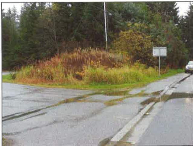
Looking eastward along Glacier Highway at TCE-12
