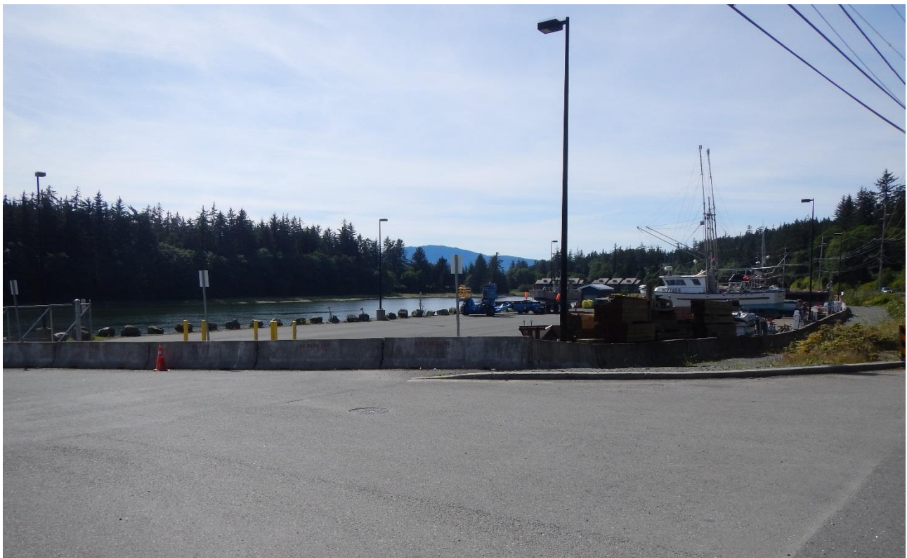
PHOTO 1 – LOOKING AT SUBJECT LEASE AREA FROM GLACIER HIGHWAY IN A WESTERLY DIRECTION.
