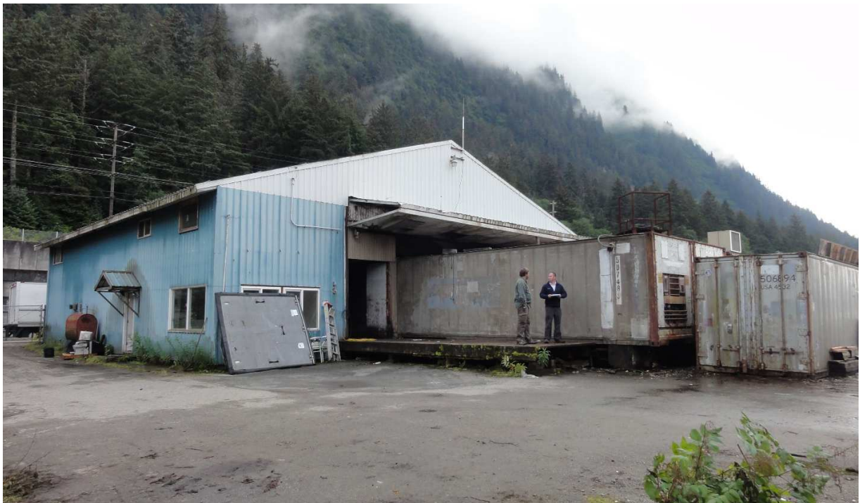
PHOTO 6 – REAR OF WAREHOUSE. (081315_12278)
