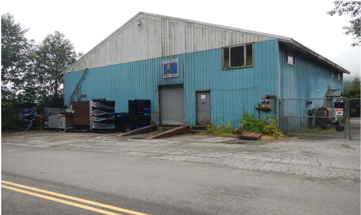
PHOTO 1 – WAREHOUSE (FORMER SEAPLANE HANGAR) AT 2601 CHANNEL DRIVE OR AS VIEWED FROM STREET. (081315_12239)
