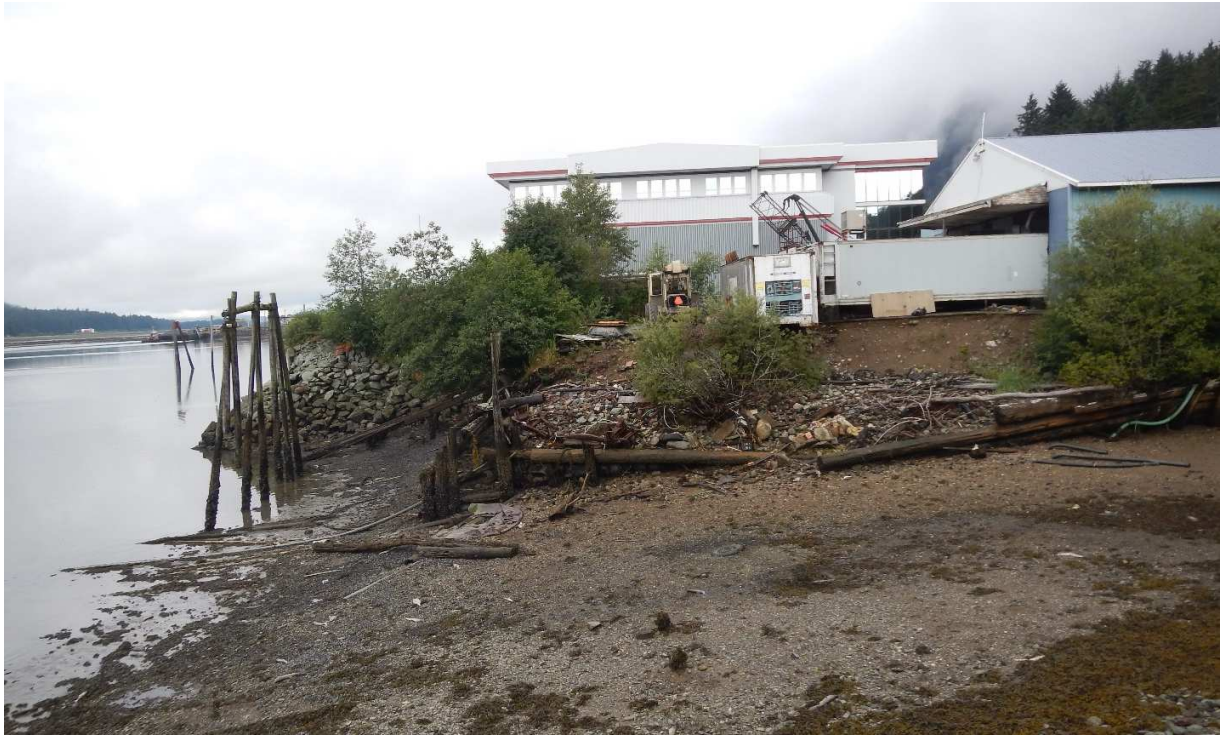
PHOTO 3 – VIEW OF SUBJECT LOOKING NORTHWEST FROM GRANT-WICK PARCELS. (081315_12254)
