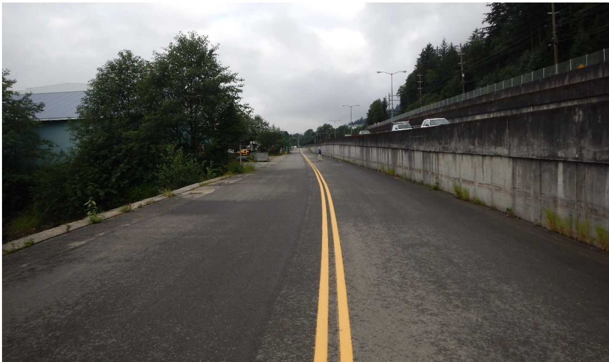
PHOTO 2 – CHANNEL DRIVE LOOKING NORTHWEST, SUBJECT PHOTO LEFT. (081315_12241)
