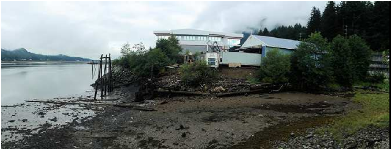
CHANNEL FLYING LEASE, WAREHOUSE AND CHANNEL DRIVE PHOTO RIGHT (081315_12270)
