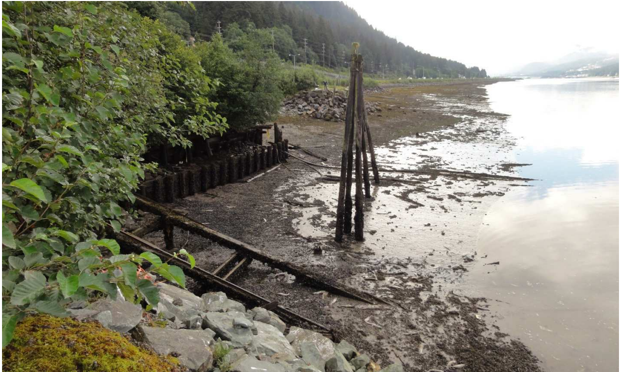
PHOTO 5 – RAMP, PILING AND SEAWALL REMNANTS ON SUBJECT PARCEL LOOKING SOUTHEAST. (081315_12273)
