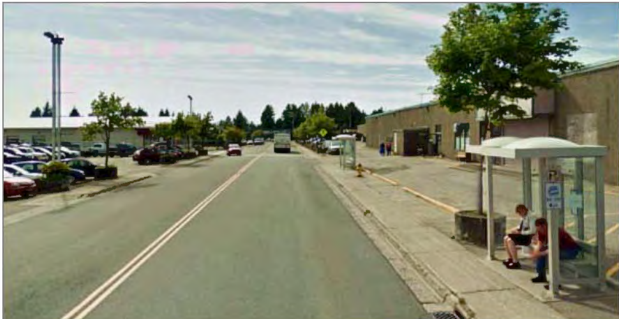
Figure 5 Nugget Mall Transfer Facility
