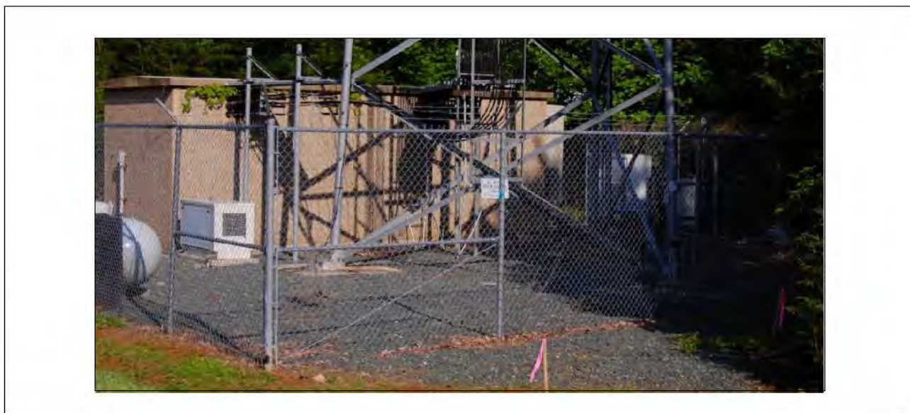
Figure 2: Example of 800 MHz Base Station
