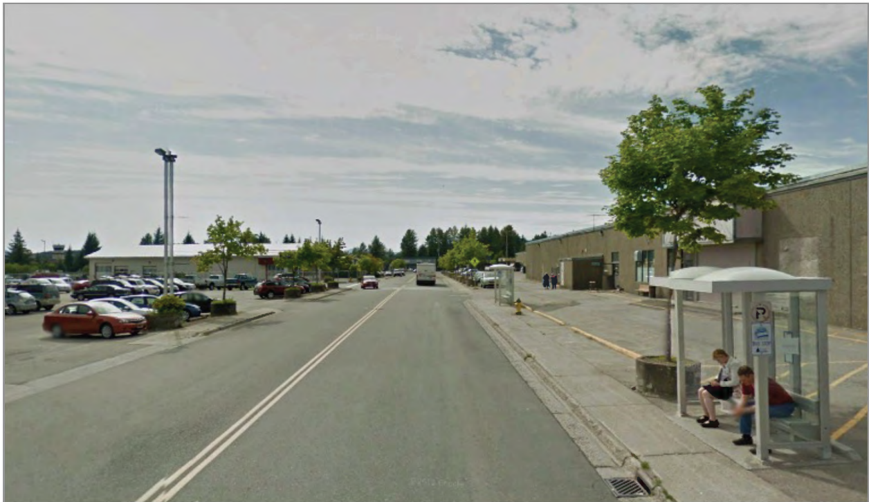
Figure 5 Nugget Mall Transfer Facility
