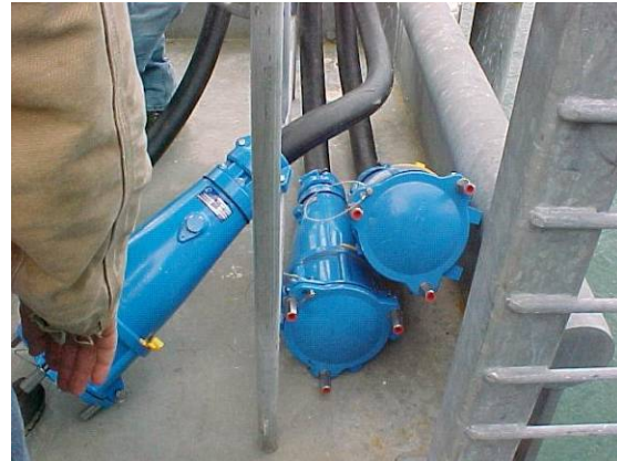
Figure 2 - Shore Tie Connectors
