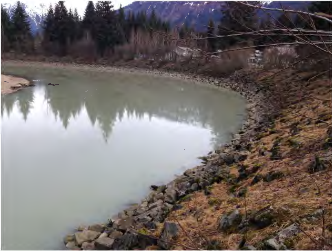
Figure 3: Existing riprap near Postal Way
