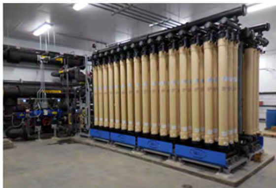
Left to right: new SC water filtration building; new microfiltration membrane units
