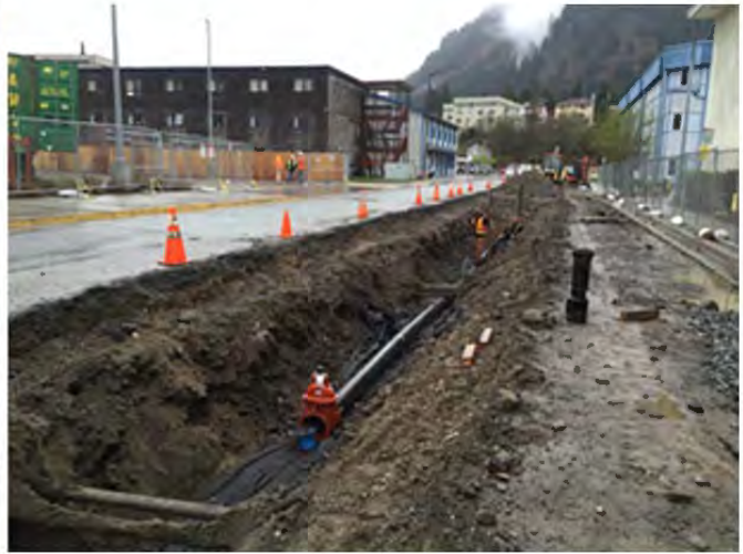
HDPE waterline installation on Whittier Street
