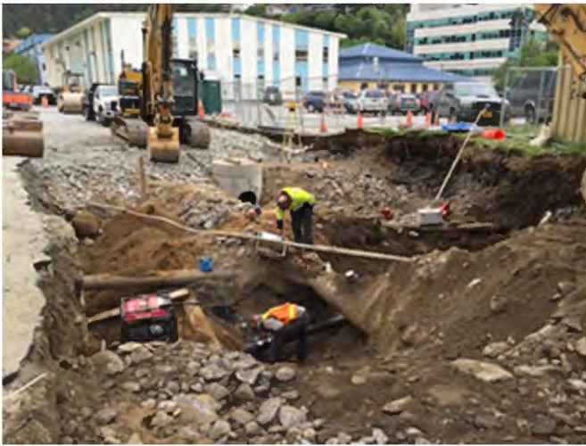
HDPE waterline installation on Whittier Street
