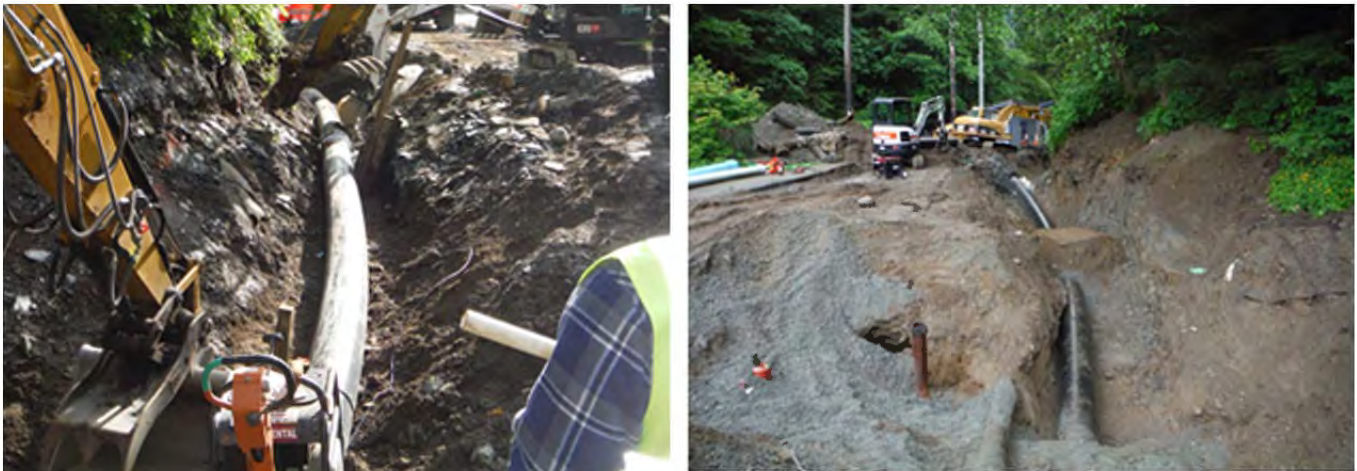
HDPE waterline installation at Cope Park
