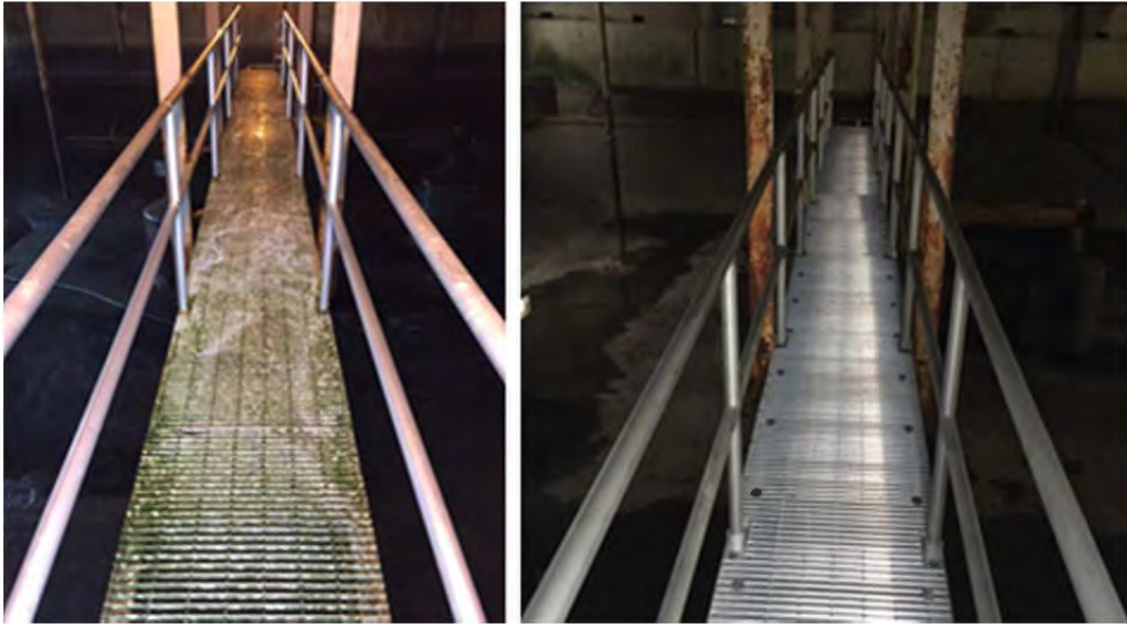
Left to right: JDTP old catwalk over digester; new calwalk and handrails
