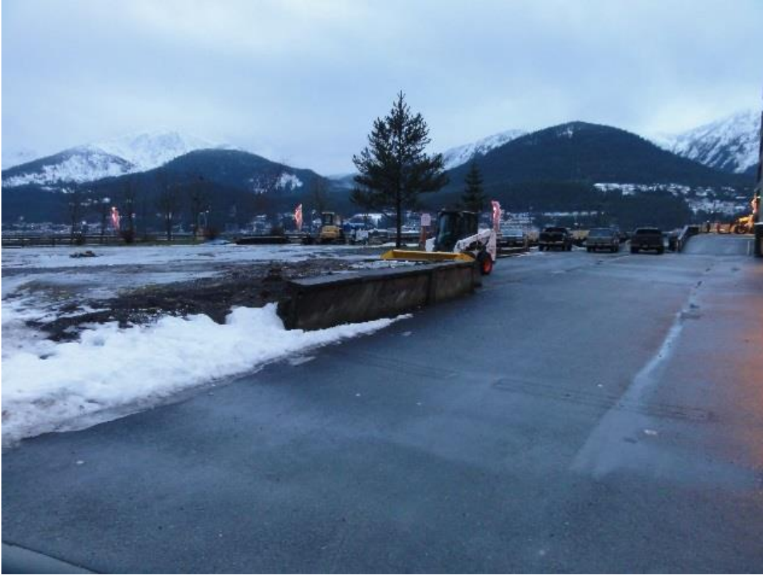
PHOTO 11 - Strip of land along north edge of Archipelago Property looking in a westerly direction toward dock. Note wooden ramp photo background right. (120417_3102)
