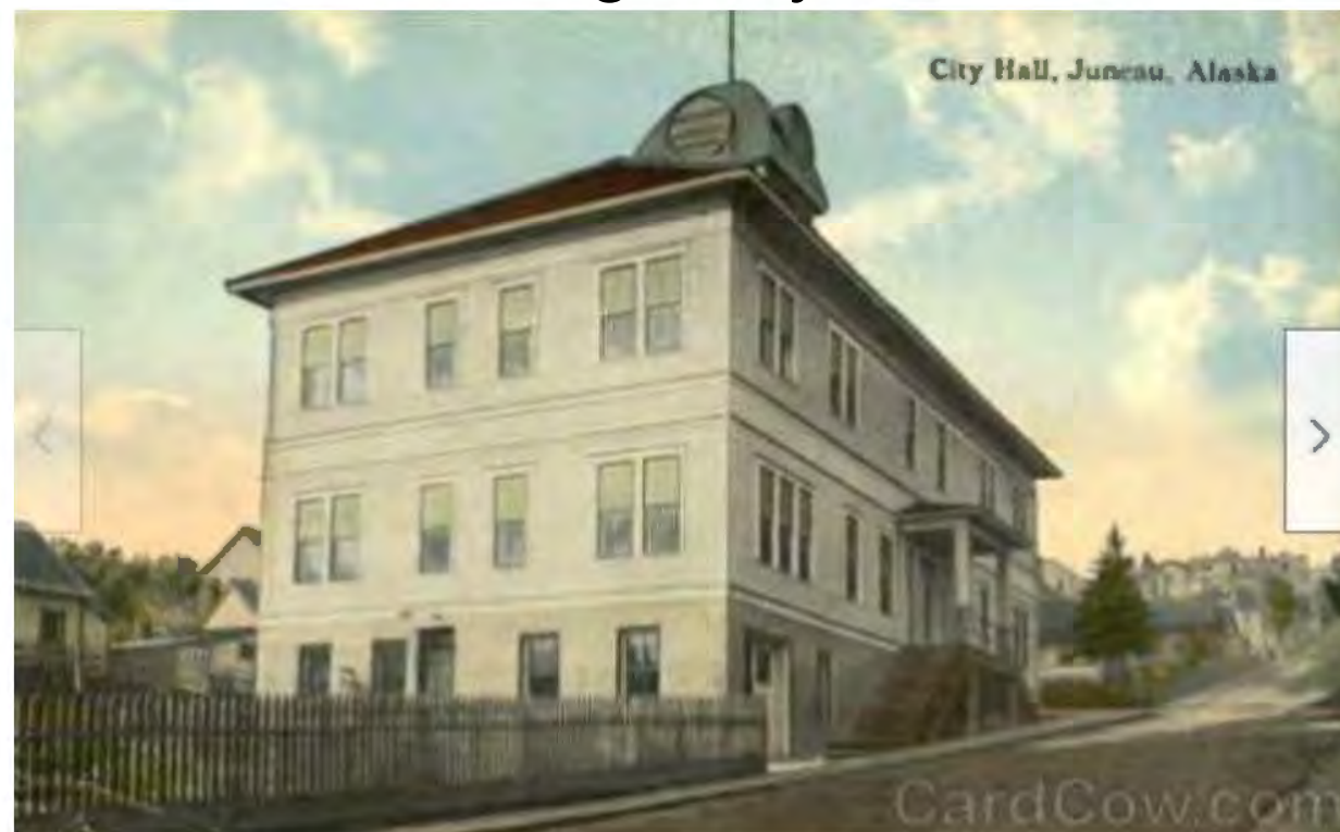
Historic Juneau City Hall
