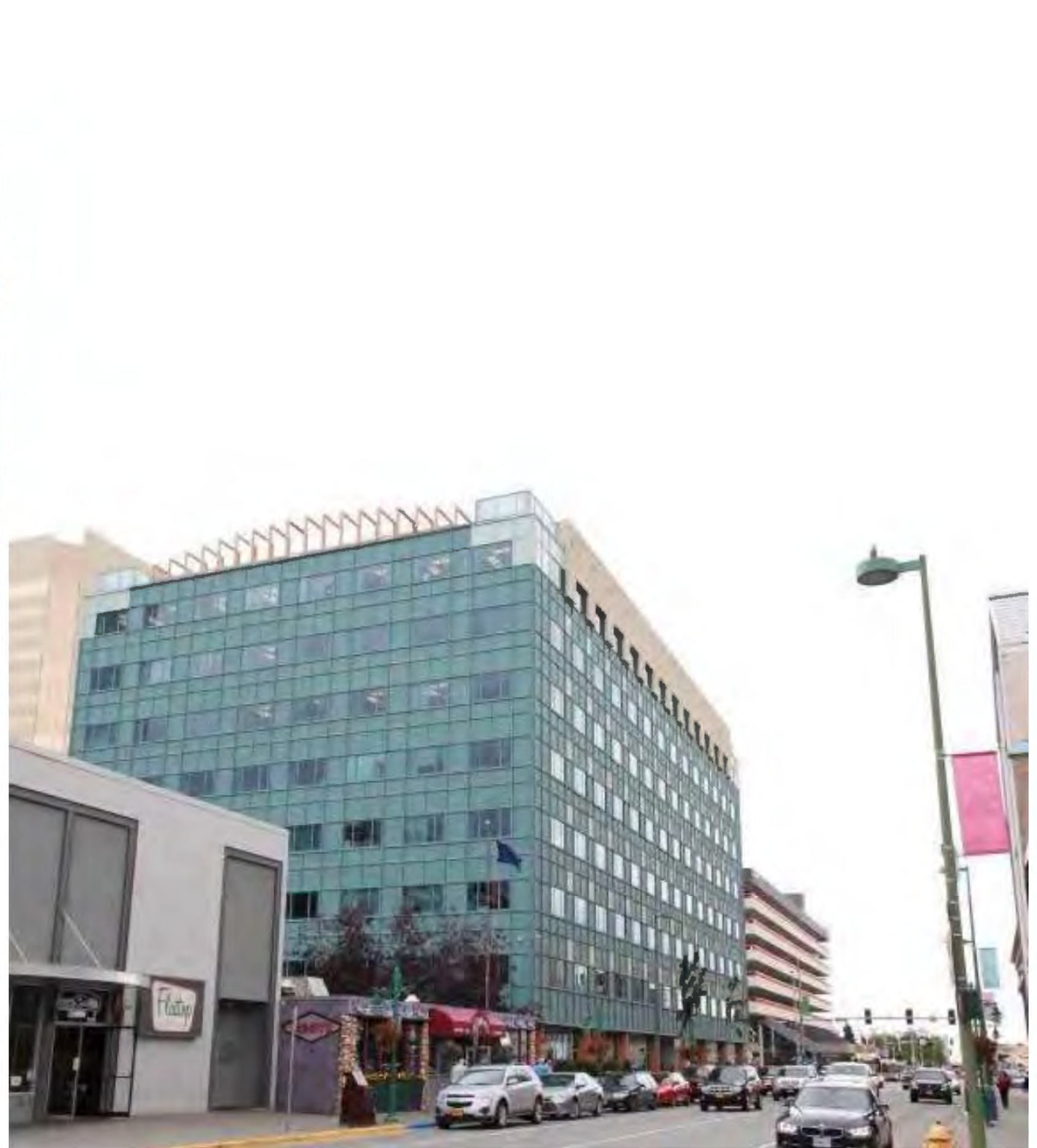
Anchorage City Hall
