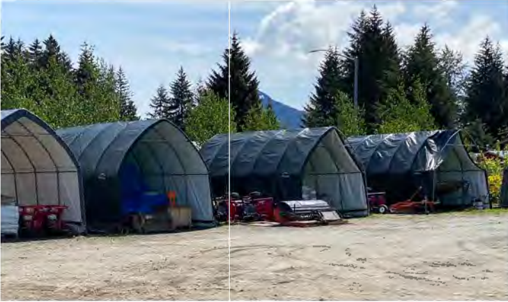
Existing temporary tents, damaged over winter
