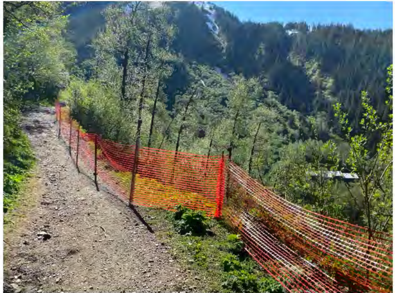
Landslide above Basin Rd. trailhead (May 2022)
