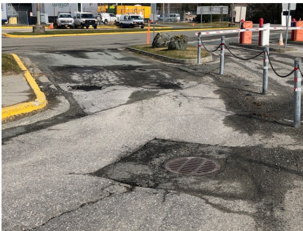
Taxi staging lot entry
