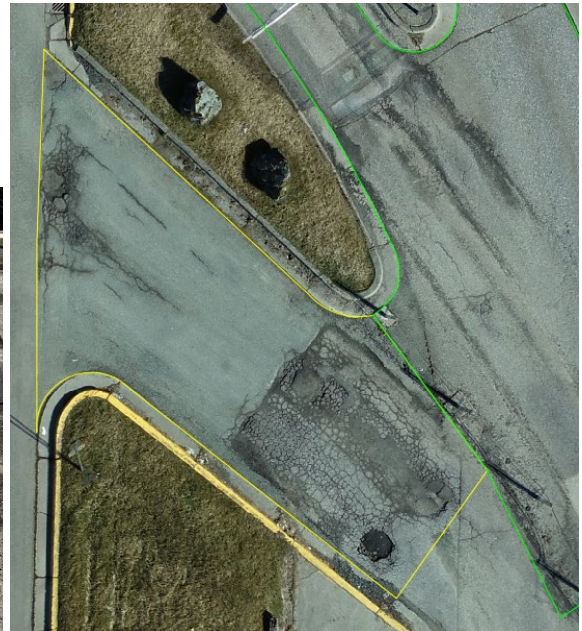
Taxi staging lot entry
