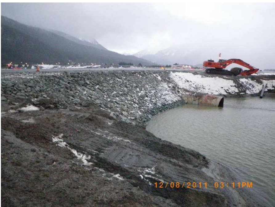
This image shows some of the rip rap slope stabilization that AIC installed at the Jordan Creek excavation site in preparation for winter shutdown.
