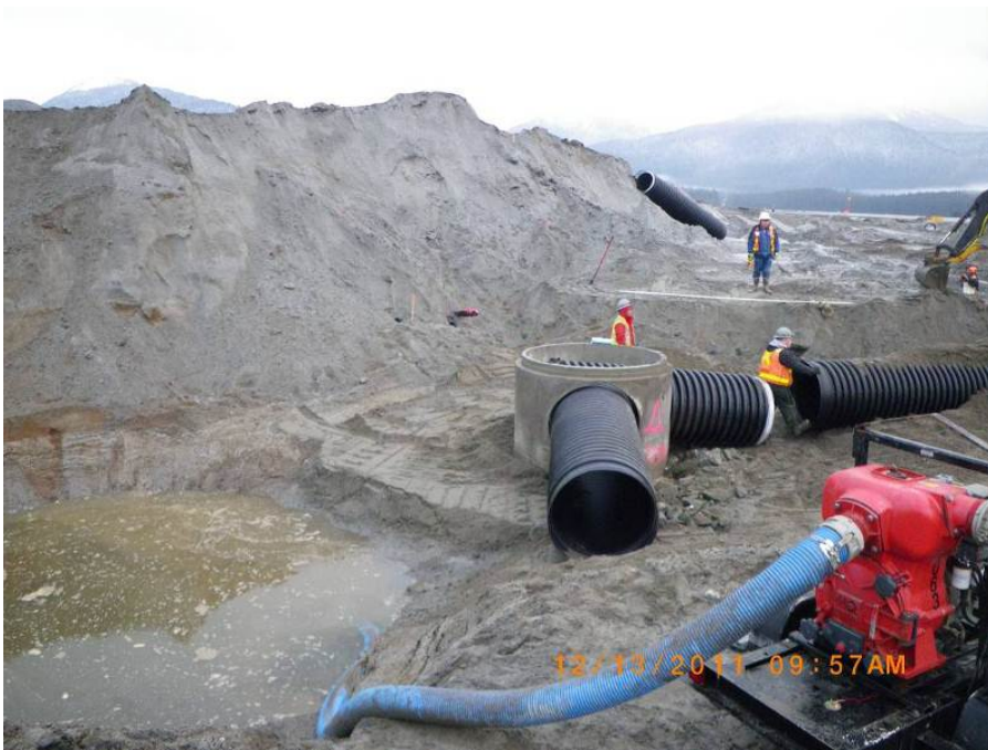
This image shows storm drain work underway in the N.E. Development area. Stockpiled dredge material is visible just beyond the new storm drain manhole.
