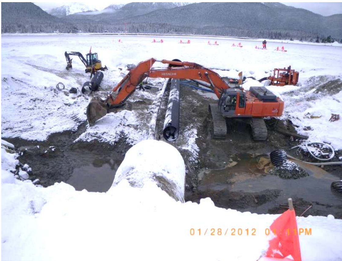
This image, taken on January 28, shows the 36" bypass culvert being installed in the infield. It will hopefully carry excess flows from Jordan Creek through the work zone without flooding the area.
