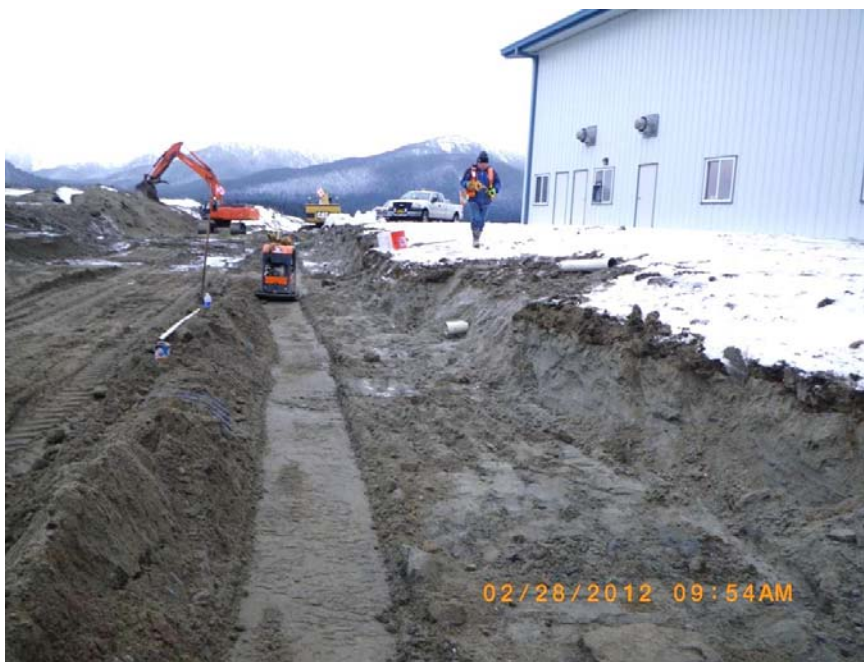
This February 28 image was taken from the edge of Yandukin Drive, looking south towards the runway. It shows compacted backfill over the newly installed storm drain system. The building to the right is the Wings of Alaska hangar. The NE Development Area is to the left.
