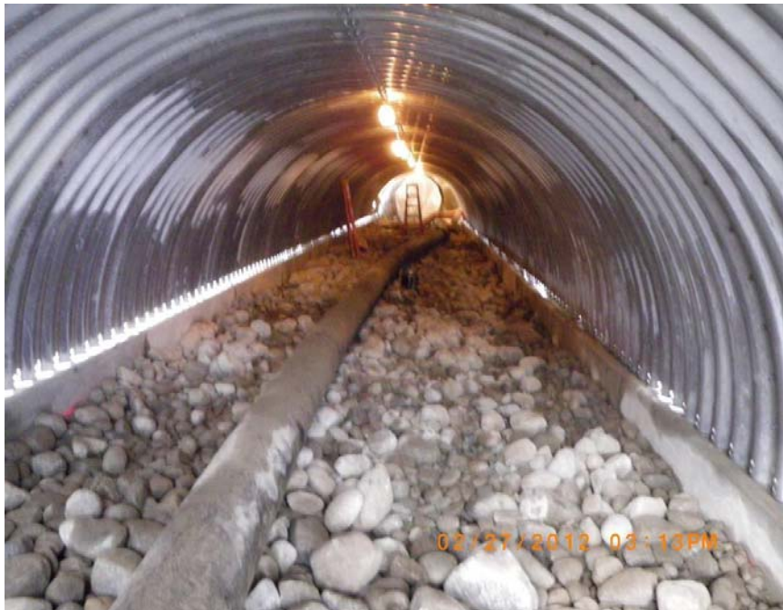
This image, also taken on February 27, shows the interior of the 14' arch culvert. Note the concrete stem walls on either side and the round river rock that will be the Jordan Creek streambed.
