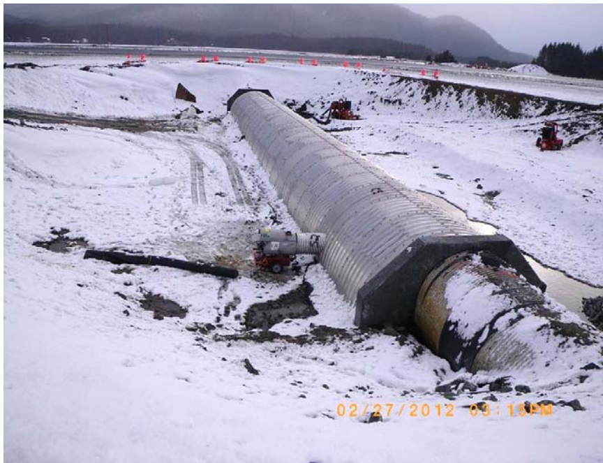
This image shows the Jordan Creek infield area on February 27. The arch pipe is in place and the following day it was grouted into the keyway along the top of the stem walls. The existing 8' round culvert beneath the taxiway is visible in the foreground; the runway is visible in the distance
