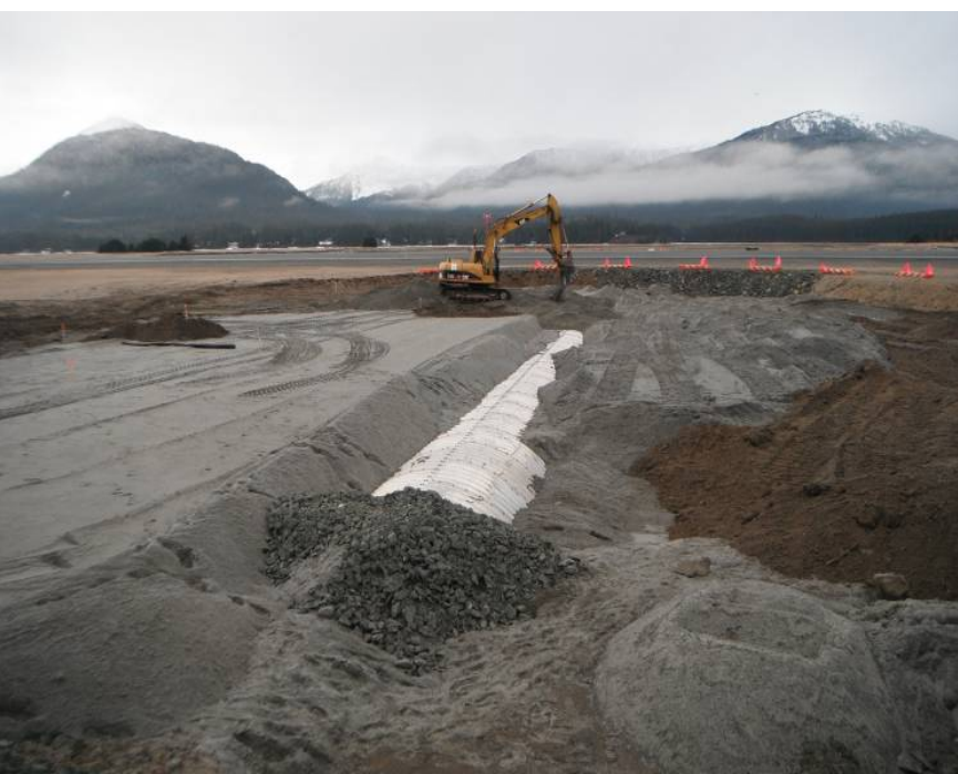
This image shows the Jordan Creek infield area on March 17. Backfill over the arch pipe is almost complete. By March 19, topsoil and grading was completed. The runway is visible in the distance.
