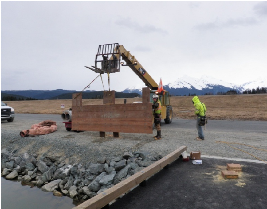
This image, taken on April 3, shows the timber face for the face of the long Ward Air loading dock. The purpose of the timber structure is to protect the Otter floats when moored at the dock.
