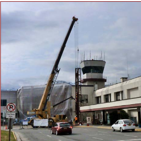
Pile driving for new canopy columns.
