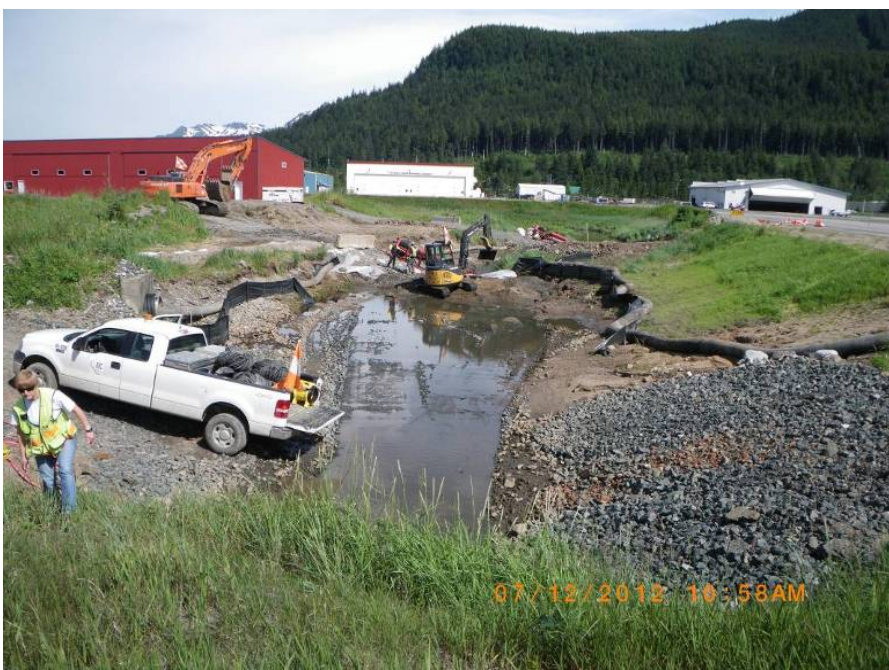
This image, taken on July 12, shows the successful water control approach for allowing work inside the Jordan Creek culvert.
