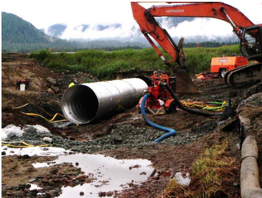
This image, taken on July 27, shows the first 40' section of culvert being positioned for installation into the existing Jordan Creek culvert. By July 29, all three sections were successfully installed. Grouting began on July 31.
