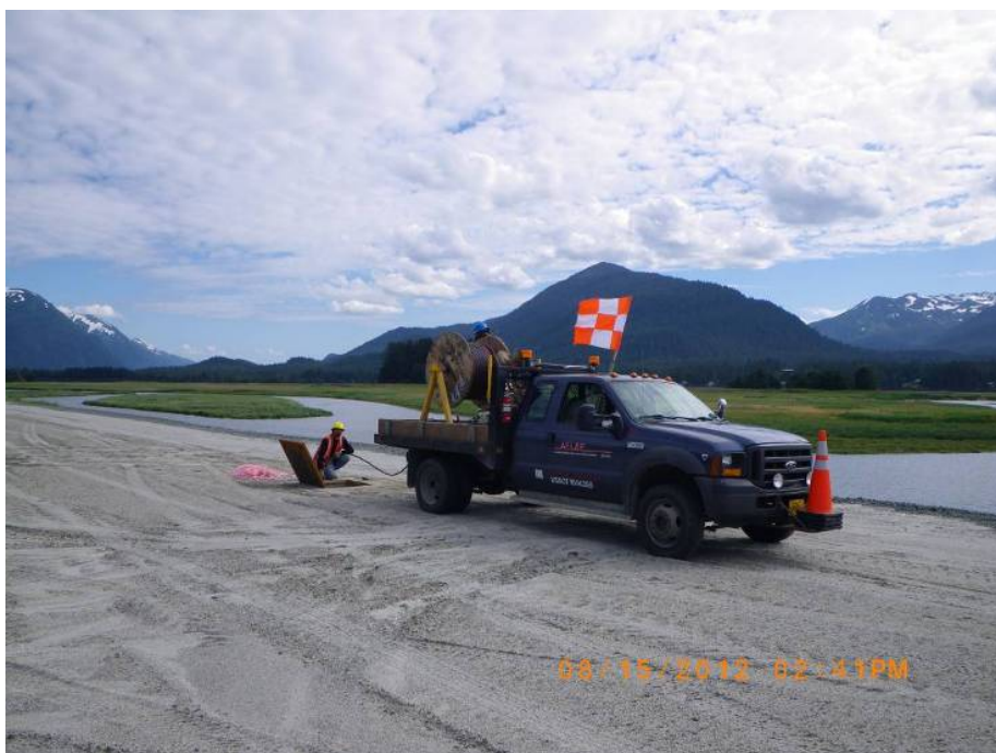
This image, taken on August 15, shows AEL&P pulling conductors for high voltage primary power that will go the east end of the runway.
