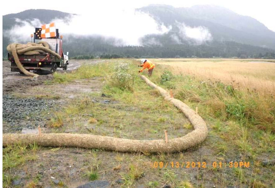
This image, taken on September 13, shows SWPPP measures being installed at the east end of the RSA.
