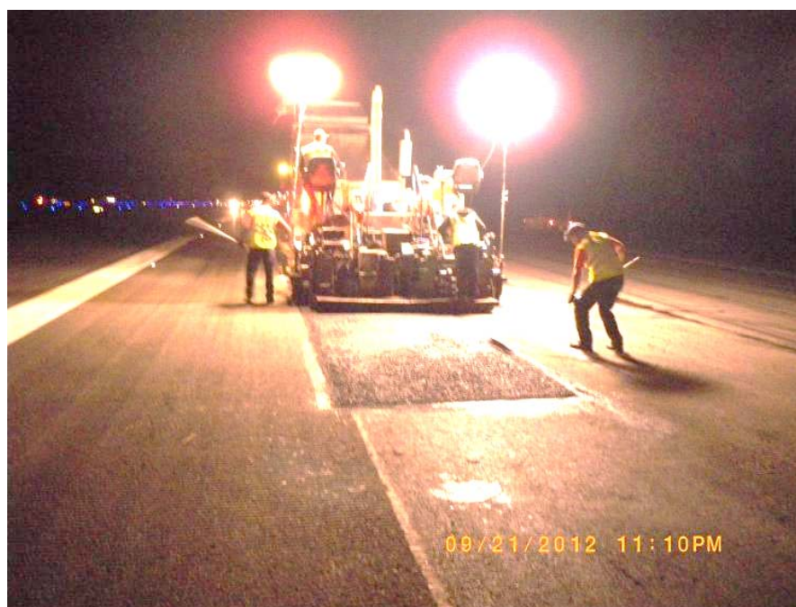
This image, taken on September 21, shows the night time operation to repair logitudinal joints on the runway.
