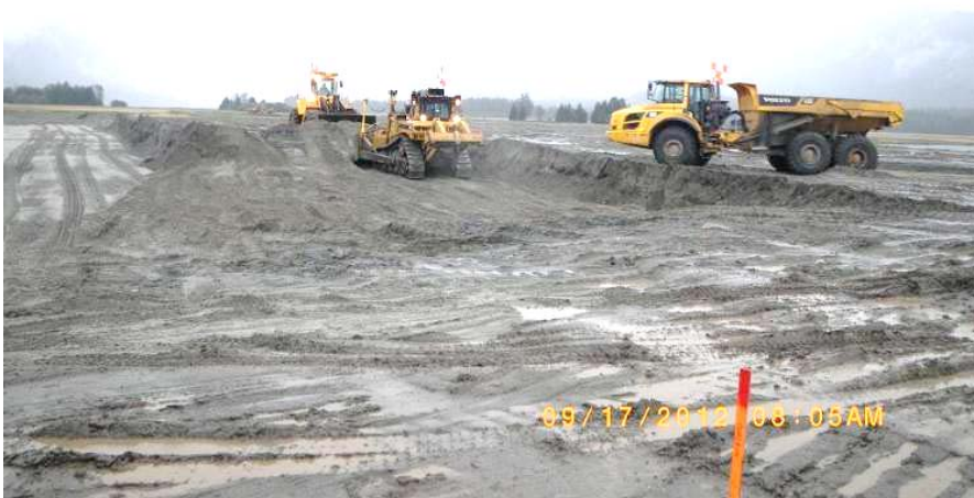
This image, taken on September 17, shows Channel Construction excavating material in preparation for the structural section for the extended runway and taxiway.
