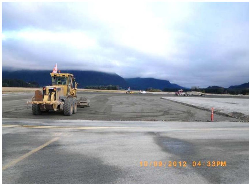
This image, taken on October 9, shows D-1 being placed for runway 26 extension.
