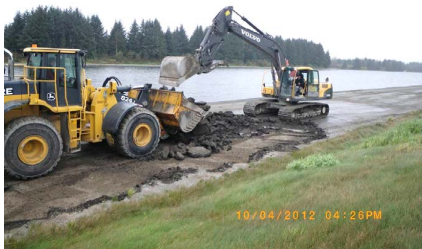
This image, taken on October 4, shows asphalt removal underway on north float plane pond road.
