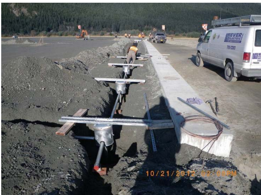
This image, taken on October 21, shows Ever Electric installing threshold lights. Also visible is the newly completed threshold bar that was installed by FAA's contractor
