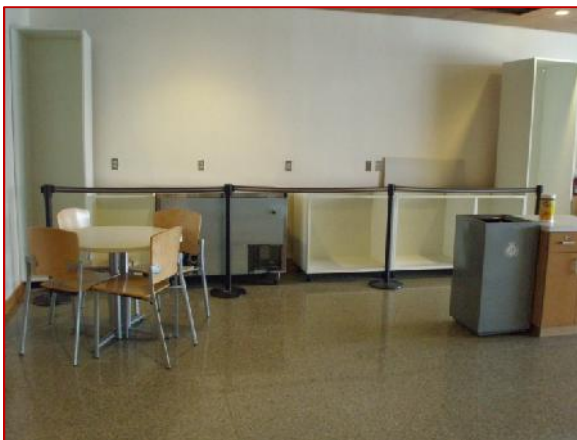
Construction underway for Departure Lounge coffee bar.
