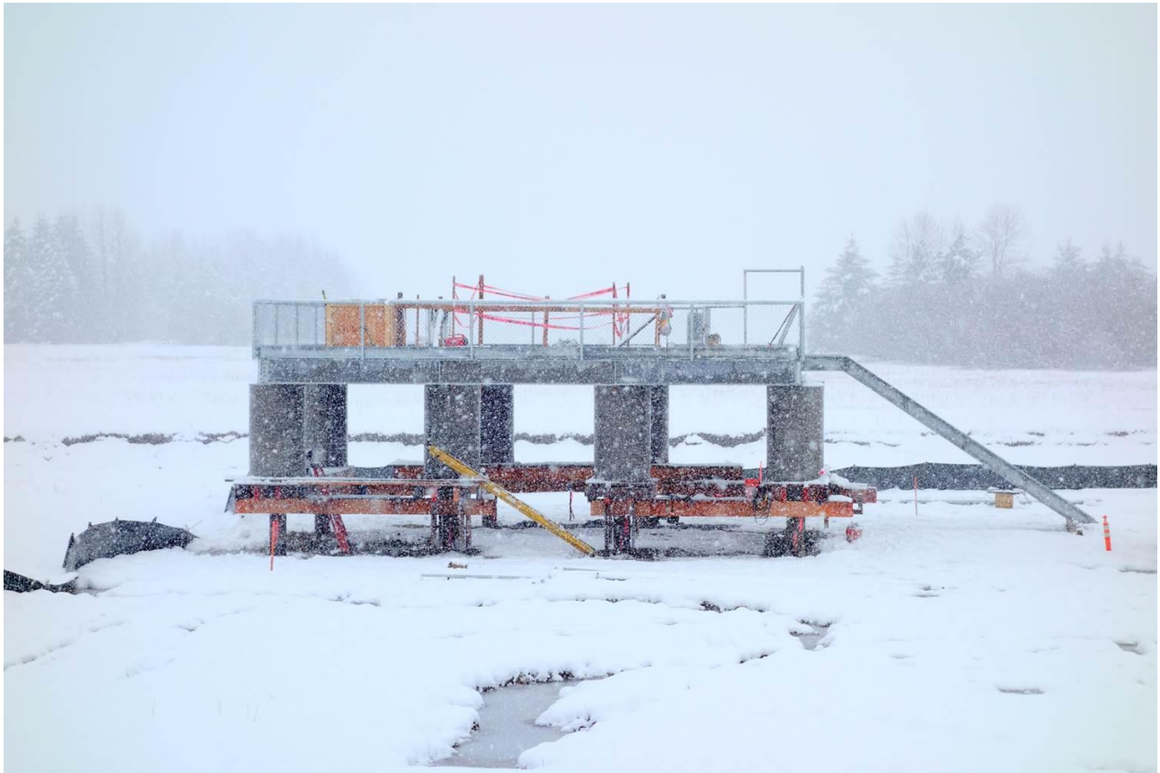
Construction of the 26 MALS platform at Station 8
