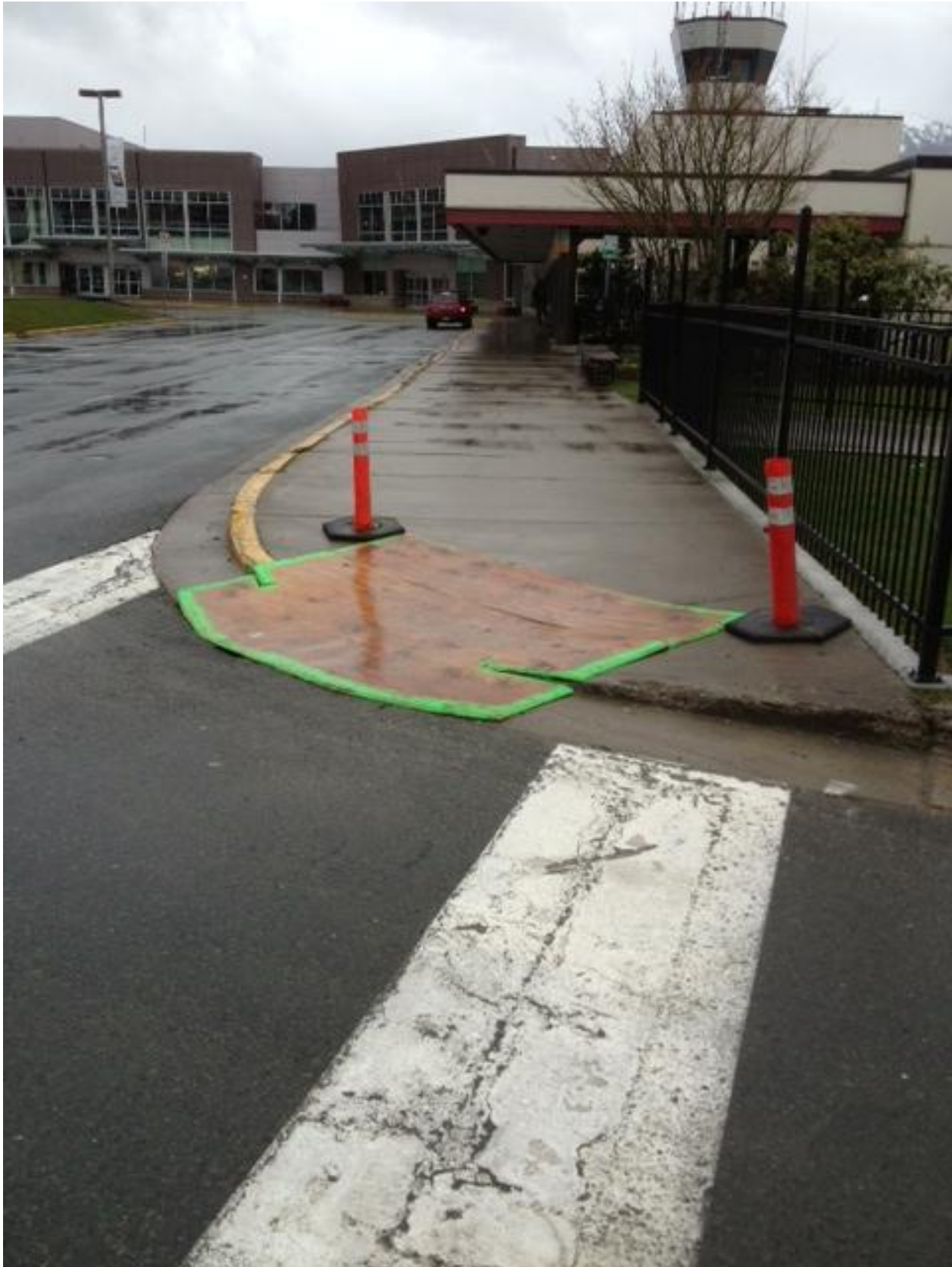
Temporary pedestrian ramp leading to the terminal.
