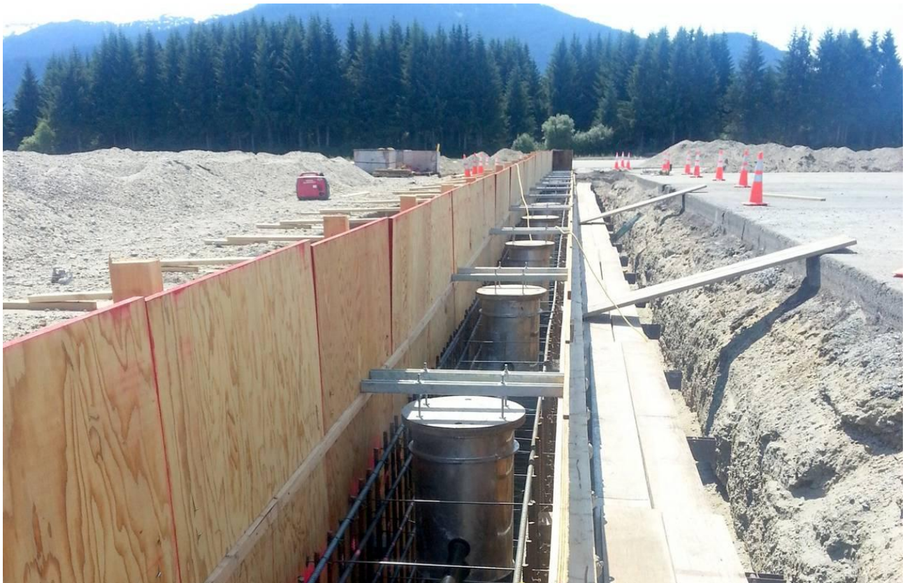
Runway 8 Threshold Installation
