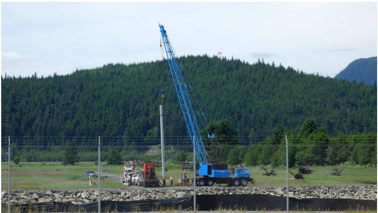
Pile Driving for the new 8 MALSR System
