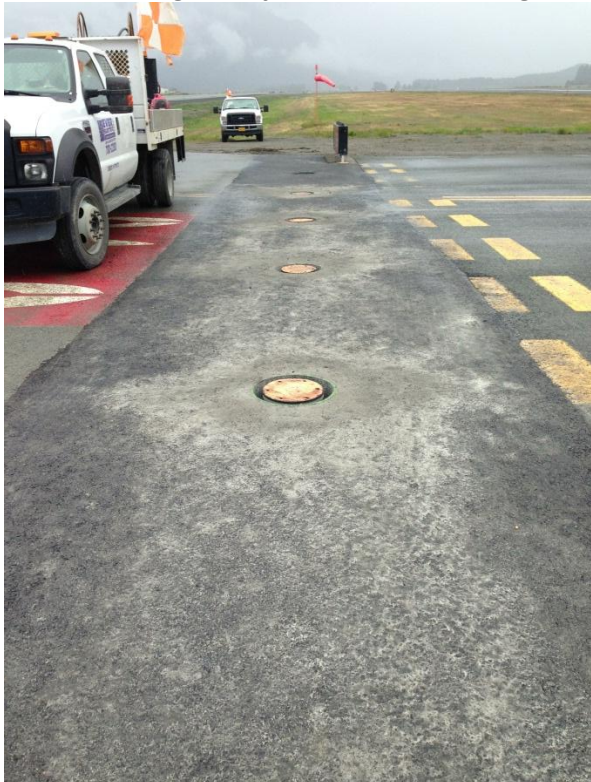
TWY F In-Pavement Runway Guard Light Installation
